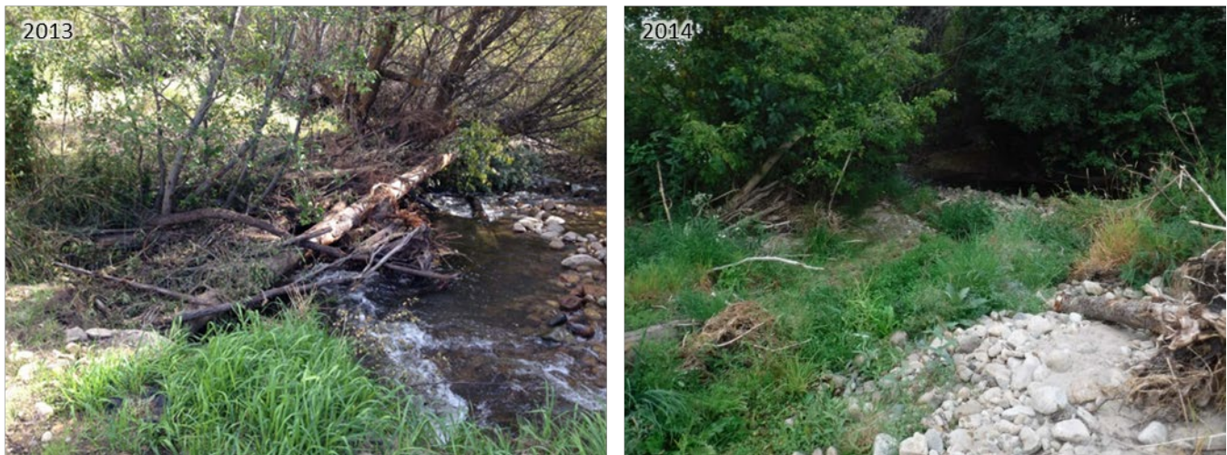
Figure 3-31. Site A looking downstream. Left: immediately post-construction (2013). Right: post-fire, post-5-year flow event (2014).
