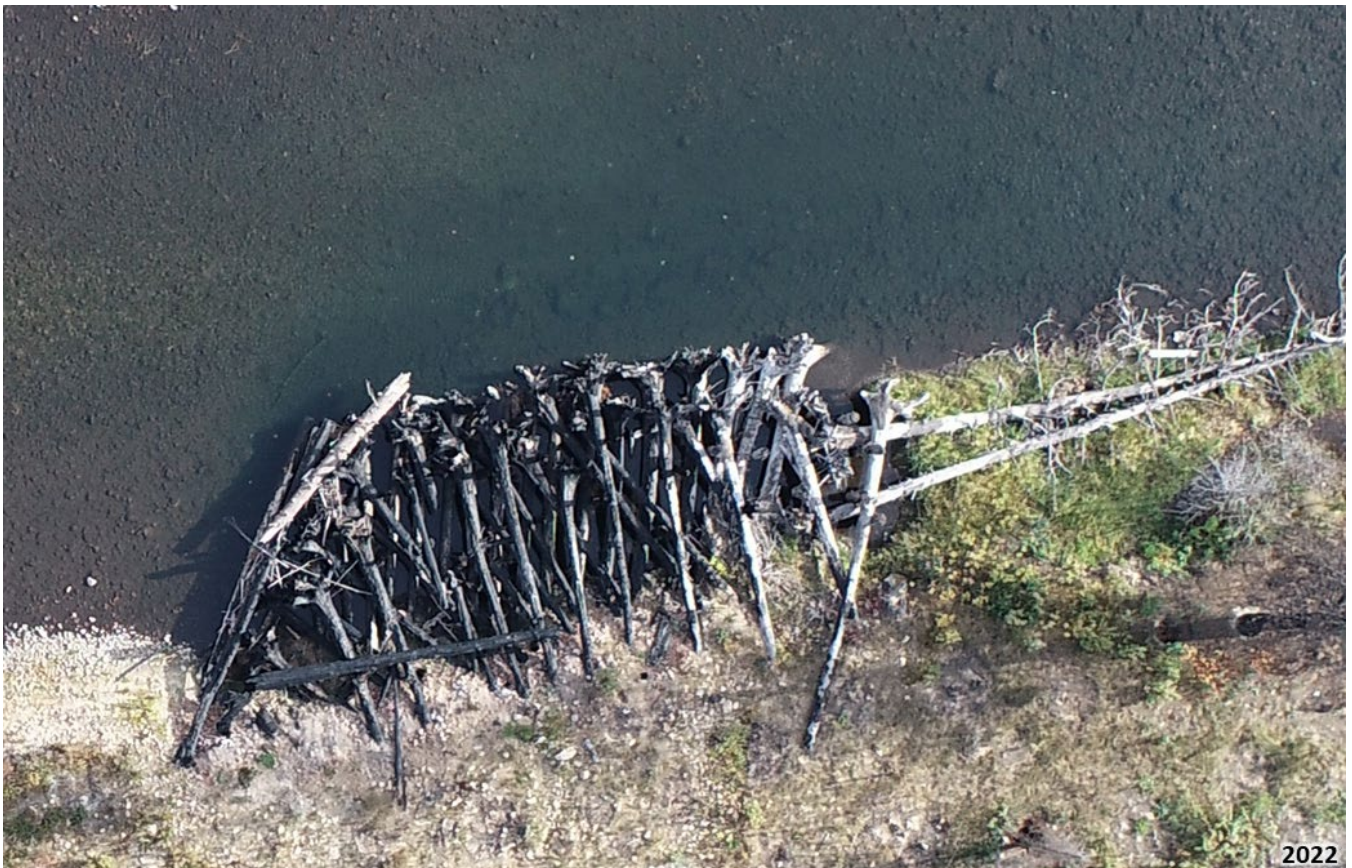
Figure 3-14. Overview of Site E post-fire. Flow is left to right.
