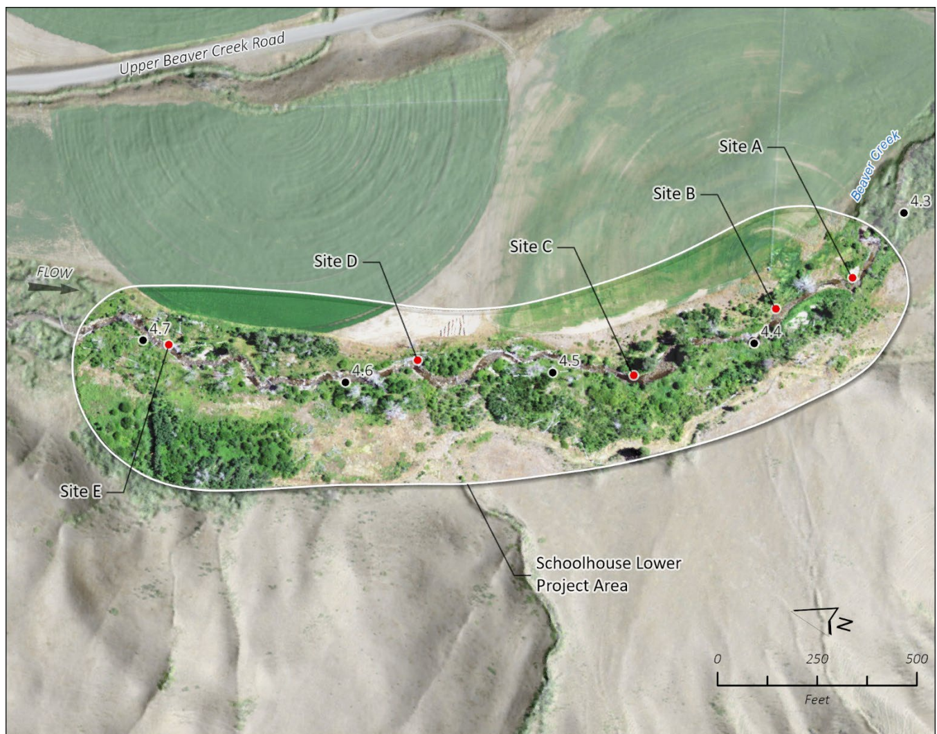
Figure 3-26. Overview of lower project area treatments.
