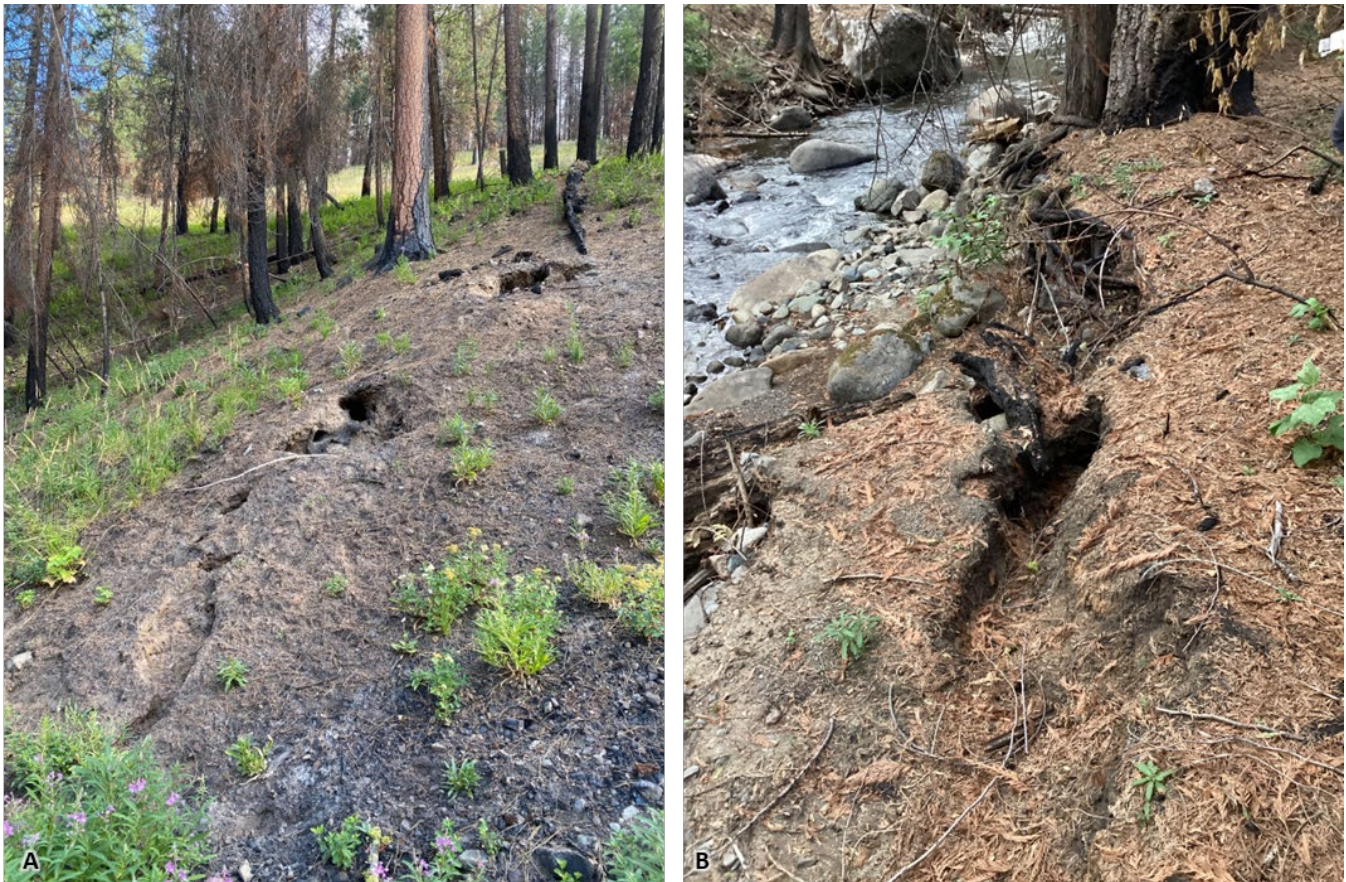
Figure 3-47. Example photos of post-fire soil erosion processes at A) burned root void collapse and piping instigating upslope rill-development on a floodplain terrace at RM 4.08; and B) destabilized bank collapse at RM 4.47. Photos collected August 11, 2022.
