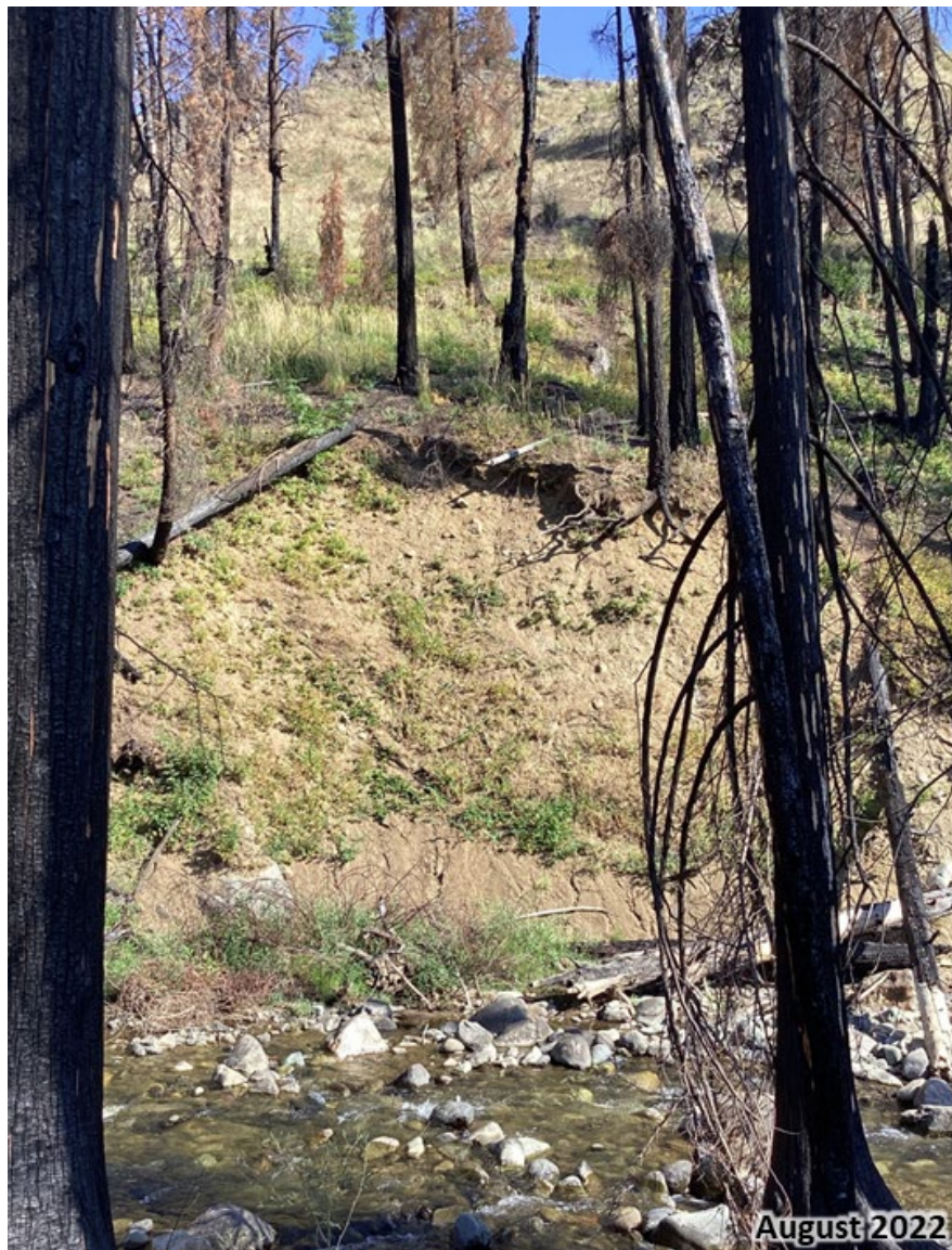
Figure 3-51. Unstable hillslope at R 3.37 on river left – contribution sediment and large wood. Photo taken August 11, 2022.
