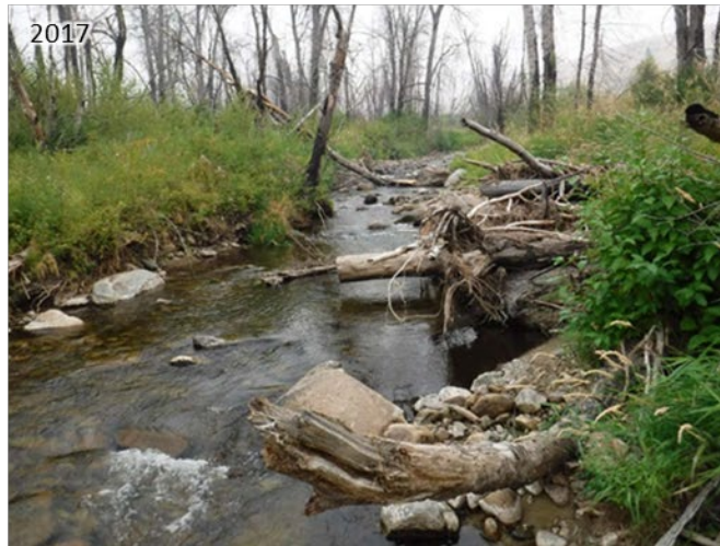
Figure 3-36. Site E looking upstream. Upper left: immediately post-construction (2013). Upper right: post-fire, post-5-year flow event (2014). Bottom: post-7.5-year flow event (2017).
